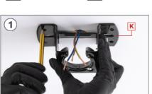
Mark on the ceiling with a pencil the 4 holes of piece **K**.
