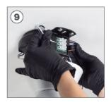
Then, you have to join the remaining wires of piece B and the line and neutral wires from your house wiring in the block terminal in piece K, as shown below.
