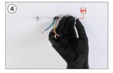
Only the thread of the screw should stick out.
