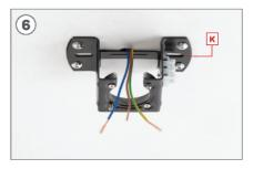
Make sure that part **K** is perfectly fixed to the ceiling and that no wires are trapped.
