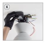
Once the wires are connected, insert piece **B** inside piece **K**, as shown in the image.
