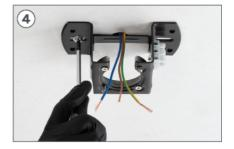
Place piece **K** and screw the fixing screws to the false ceiling.
