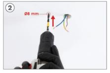
With the help of a drill, make the two corresponding holes with an Ø8 mm drill bit.
