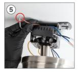
Connect the LINE (L) wire from the ceiling to the white wire from piece  ${\bf B}.$
