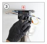
Insert part  ${\bf B}$  in the groove of piece  ${\bf K}$ . Check that all wires are correctly placed without being trapped.
