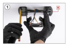
Mark on the ceiling with a pencil the 4 holes of piece **K**.
