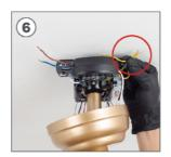
Select and connect all the grounding wires together, including the one from your own house wiring.
