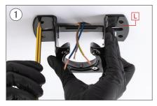
Mark on the ceiling with a pencil the 4 holes of piece  ${\bf L}.$
