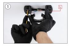
Mark on the ceiling with a pencil the 2 central holes of piece l, using the same piece as a guide.
