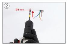
With the help of a drill, make the two corresponding holes with an  $\emptyset 8$  mm drill bit.
