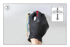
Insert the fixing screws into the holes and make sure the lever opens.
