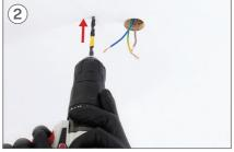
If necessary, depending on the type of ceiling, you will need to use a drill to make the hole in the wood.
