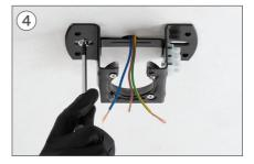
Place piece L and screw the fixing screws to the false ceiling.
