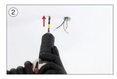
With the help of a drill, make the two corresponding holes.
