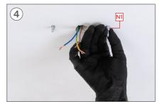
Only the thread of the screw should stick out.
