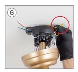
Select and connect all the grounding wires together, including the one from your own house wiring.
