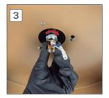
Carefully insert the fan wires inside piece S and take them out through the large side hole of this piece. Then screw piece S and check that it remains securely attached to the fan.
