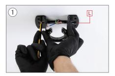
Mark on the ceiling with a pencil the 2 central holes using piece L as a guide.
