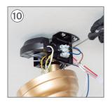
Connect the N wire from the driver with the neutral wire from your house wiring.
