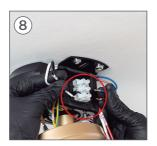
Then, you have to join the remaining wires of piece B and the line and neutral wires from your house wiring in the block terminal in piece L, as shown below.
